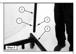
6 Insert the Right Hand Swing Arm Post Assembly (6) into the right Outer Tube on the right side of the Storage Cart Frame (8).
